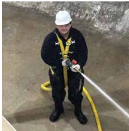
TM Rural Water District Anthony Hanisch, Apprentice Jason Krumbach, Mentor
